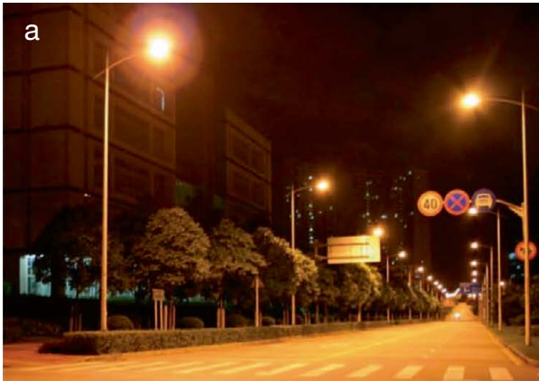
Figures 2 (a & b): New LED street lights (b) consume about 50% less energy than HP-sodium lamps (a) while providing a CRI of 80 and more homogeneous illumination. This leads to better visibility and therefore, a higher safety level (Credits: Osram)
