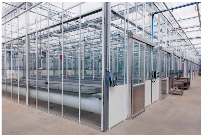
Figure 5: Research facility in Germany with cooling and heating capabilities per test cell
