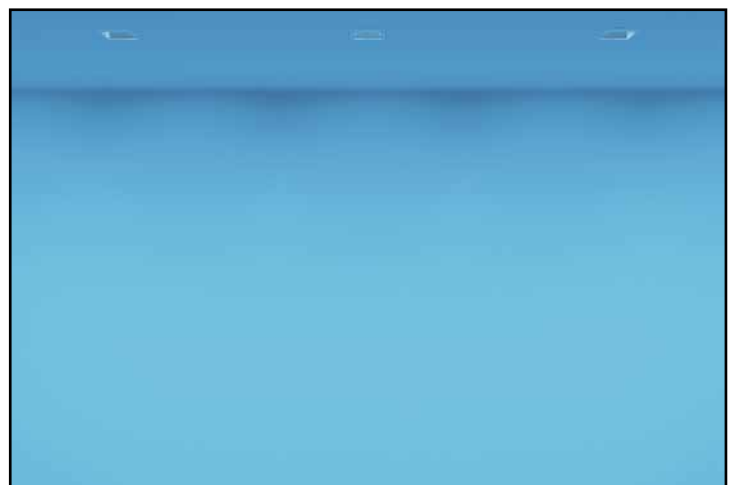
Fig. 6: Coloured wallwashing with colour compensated Quadra varychrome LED luminaire
