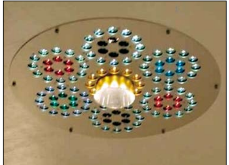
LED downlight (combined with halogen lamp for adjustable ambient lighting)
