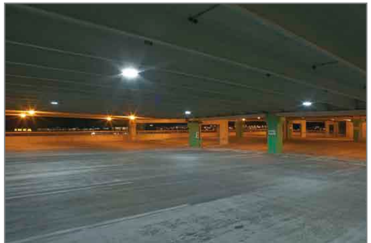
Parking ramp with Beta LED luminaires
