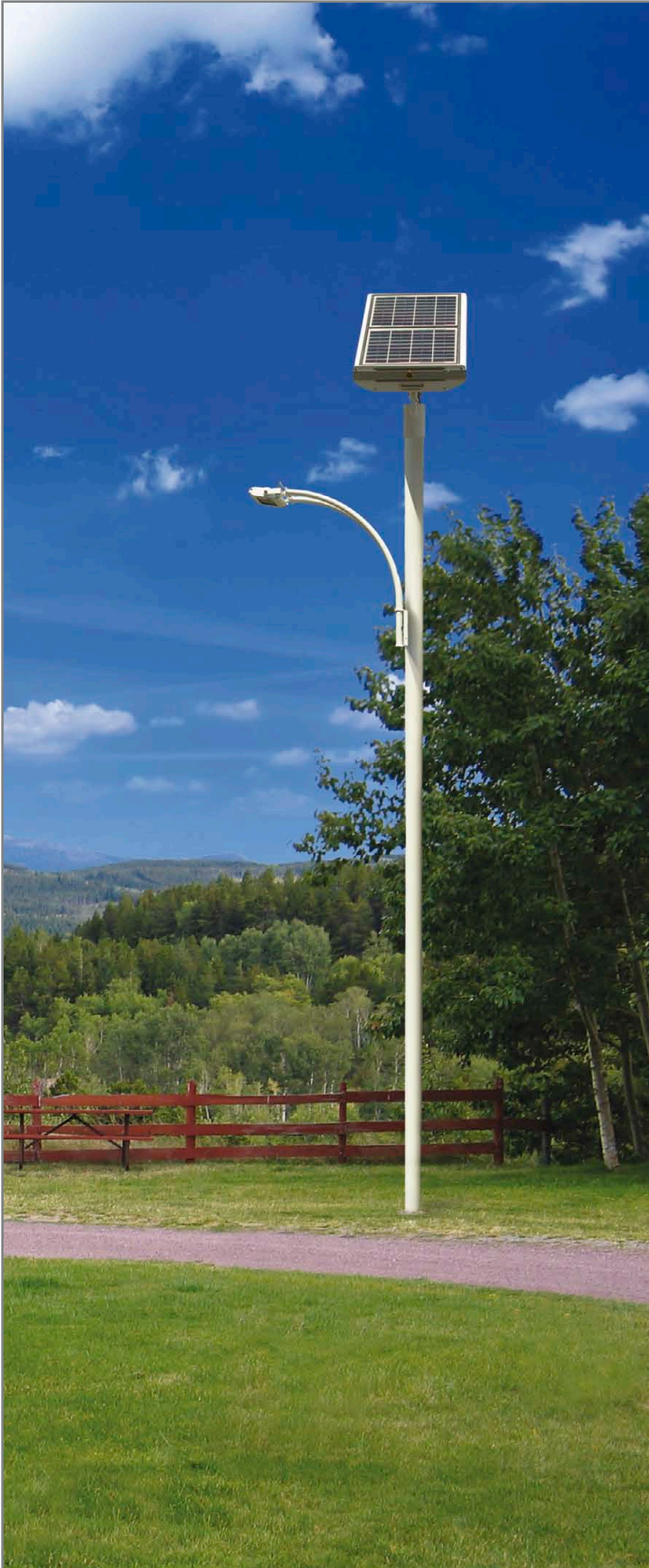
Figure 2: Area lighting in parks is one domain, where the combination of solar technology and LED technology is today's best solution
