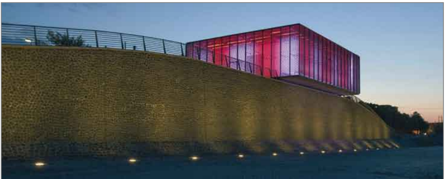
The pleasing daytime look of the high-water pumping station is only topped by the 'wow factor' that nightfall brings.
