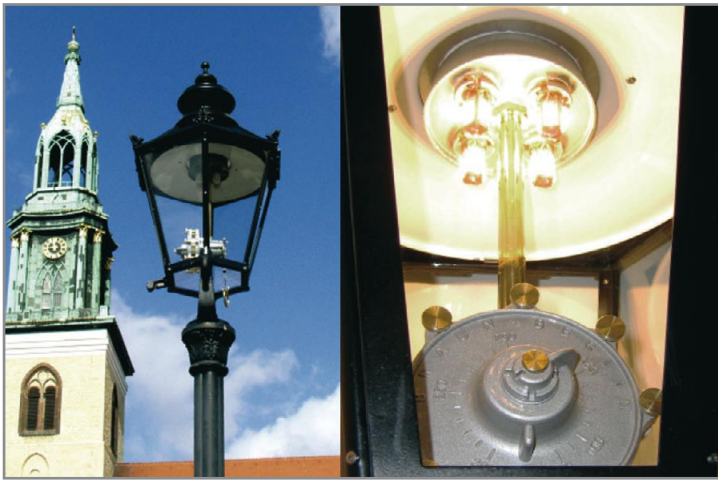
New LED module fits old gaslight form factor.
